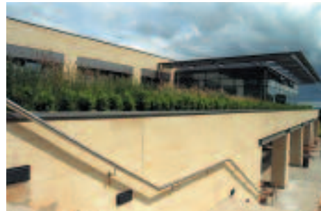
Pic: Wessex Water, Bath. Planting on a 'green' roof provides a habitat for wildlife.
